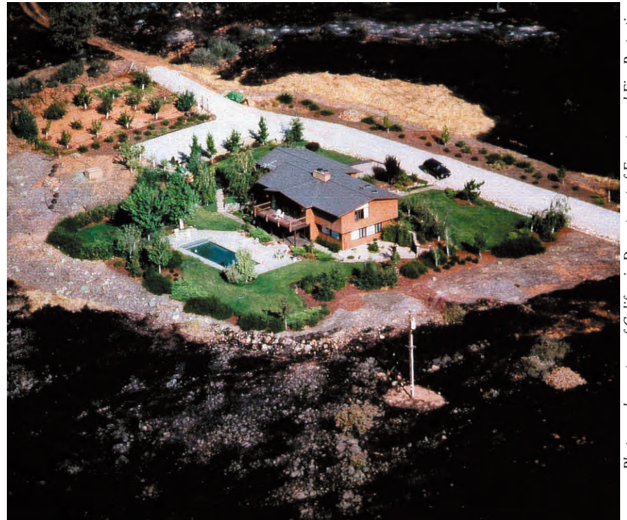
The pre-fire activities implemented by this homeowner included a green and well maintained landscape, reduction of wildland vegetation around the perimeter of the property, a fire resistant roof, and a good access road with a turnaround area. The charred surroundings of the home show that these pre-fire activities effectively protected it when wildfire hit.
